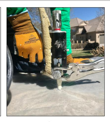
Total concrete tear out and replacement can be expensive. So can injury and liability issues when it comes to trip hazards and uneven sections of concrete that have sunk or cracked. Geotechnical polyurethane foam products are engineered to lift and void fill beneath concrete sections and save on expensive concrete replacement.
